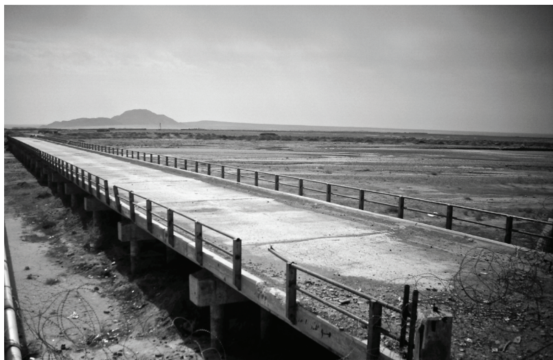
Arghestan Bridge, Kandahar province
